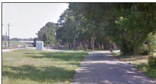
View north of the end of N. Travis St.
