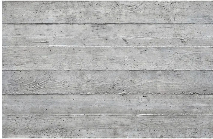
BOARD FORM CONCRETE
